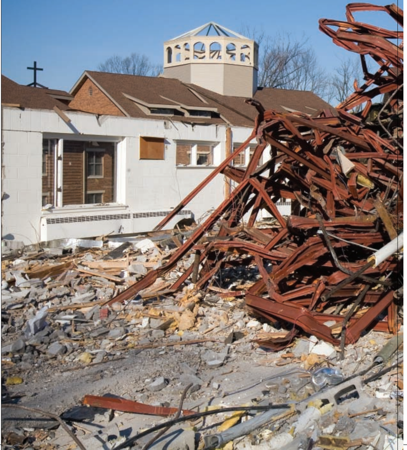
OLD MAKES WAY FOR NEW AS LENIHAN HALL IS DEMOLISHED TO CLEAR ROOM FOR THE SIENA RESIDENCE-HALL COMPLEX. STORY, PAGE 38 PHOTO BY GEOFF OLIVER BUGBEE
